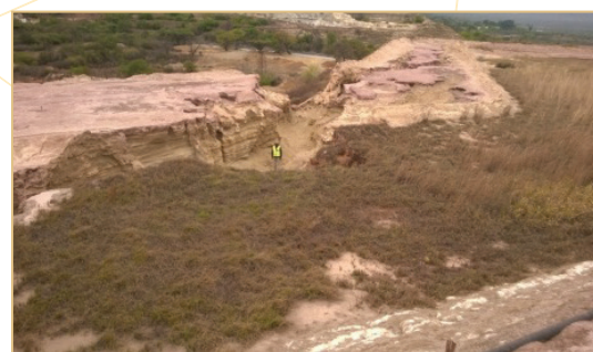
Deep gully erosion along the berms of an old tailings dam wall, Fairview mine, Barberton, Mpumalanga Province.
