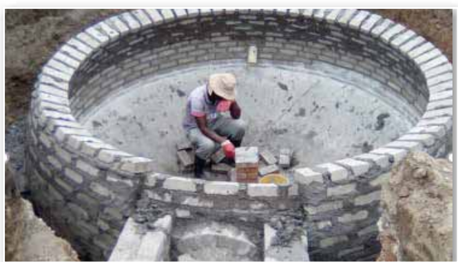
12 m 3 brick biogas digester.
