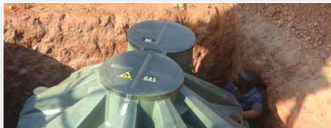
6m 3 pre-fabricated biogas digester.
