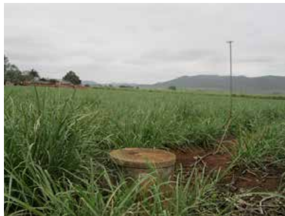
Maintenance manholes for a sub-surface drainage system.
