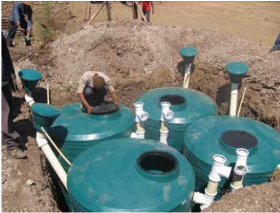
Installing a biogas digester
