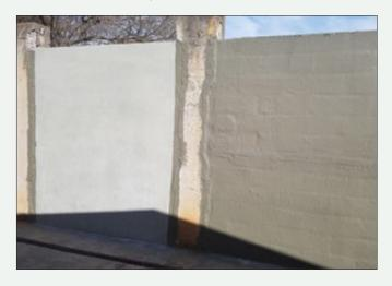
The system is intended for use in repairing and waterproofing cracked walls. It comprise a combination of high strength cementitious/copolymer modified mortar and Durox Texgrid N10.
