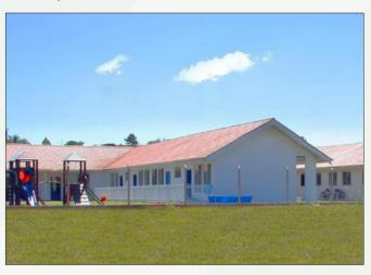
The superstructure walls are constructed of interlocking UV-resistant Polyvinyl-chloride (PVC) modules filled with concrete.
