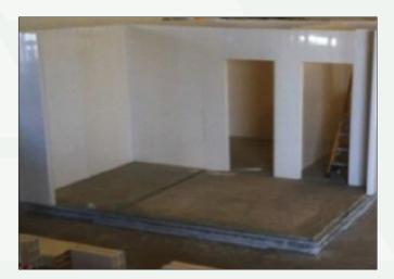
The system is for single-storey buildings and utilizes factory produced Wood Plastic Composite (WPC) extruded hollow core polymer panels (Luxwood panels) clad with Polex Board (calcium silicate board with fibres) on both sides.
