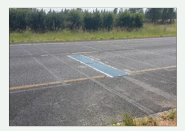
The system consists of a dual intrusive loop, BOSVARK traffic logger, Off-scale hit sensors (OS), dual ZCS-30 bending plate sensor, battery, Colseal or similar approved sealant and 3G modem that downloads data.
