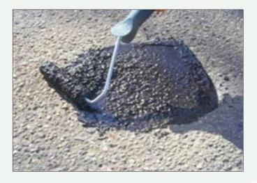
Degafill Pothole Mix is for the repair of Type 1 potholes in asphalt and concrete substrates in all regions of South Africa.
