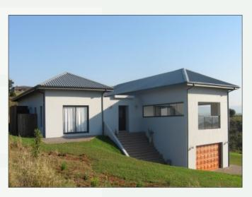
The system is a timber frame structure consisting of timber lattice beams (Eco Beams) as vertical and horizontal studs and wall plates with sandbags as infill material.
