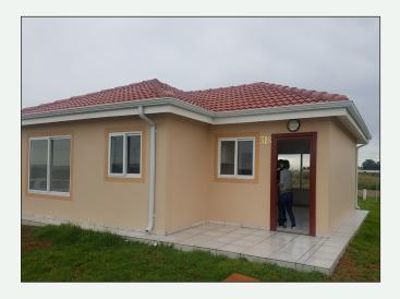
The system is for construction of single-storey structures that comprise a concrete foundation, ground-floor slab, precast concrete wall panels and a timber roof.
