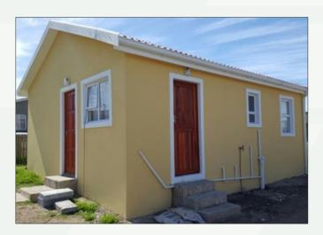
Walls are erected of factory produced light-weight masonry concrete blocks, comprising a mixture of Expanded Polystyrene (EPS) beads, cement, water and additives. blocks have a minimum compressive strength of 3 MPa.
