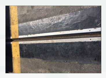
The bridge deck joint is a single rubber seal fixed between two aluminium claw brackets encased in Flexicon elastomeric concrete.
