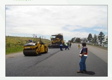
The system is laid with a nominal compacted thickness of between 10 mm and 20 mm. The product consists of an open-graded asphalt placed on a film of NOVATACK tack coat by a self-priming paver. The function of the tack coat is to seal the existing surface and to ensure a high tensile bonding between the NOVACHIP mix and the existing surface.
