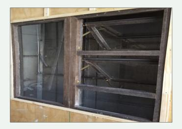
The window frame comprise window head, jambs, sill, mullions and sash profiles manufactured from an extruded heterogeneous blend of impure recycled plastic, reinforced with cellulosic fibres.
