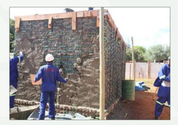
The system is for single storey buildings and utilises fishnets and PET bottles. The foundations are conventional concrete strip footing with foundation-wall and plinth constructed of only the 2 litre PET bottles.
