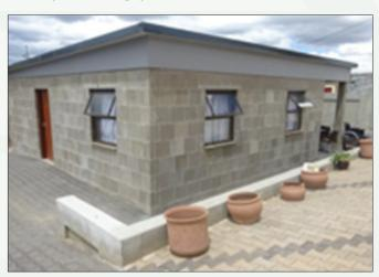
The system utilizes polymer concrete blocks that are assembled on site.
