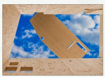
The system is for single- and double-storey structures and utilizes factory produced wall, suspended floor decking and roof panels. Foundations and surface beds are conventional and designed by a professional engineer or approved competent person.
